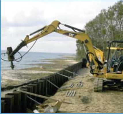
Steel Sheet Pile
