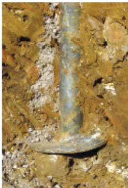
Cutaway close up of drive end bearing on shallow rock stratum
