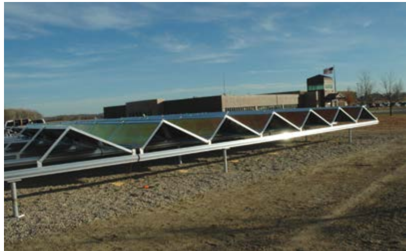
Contractor budgeted 7 days with 2 men for pier installation. Installed in 2 days.
