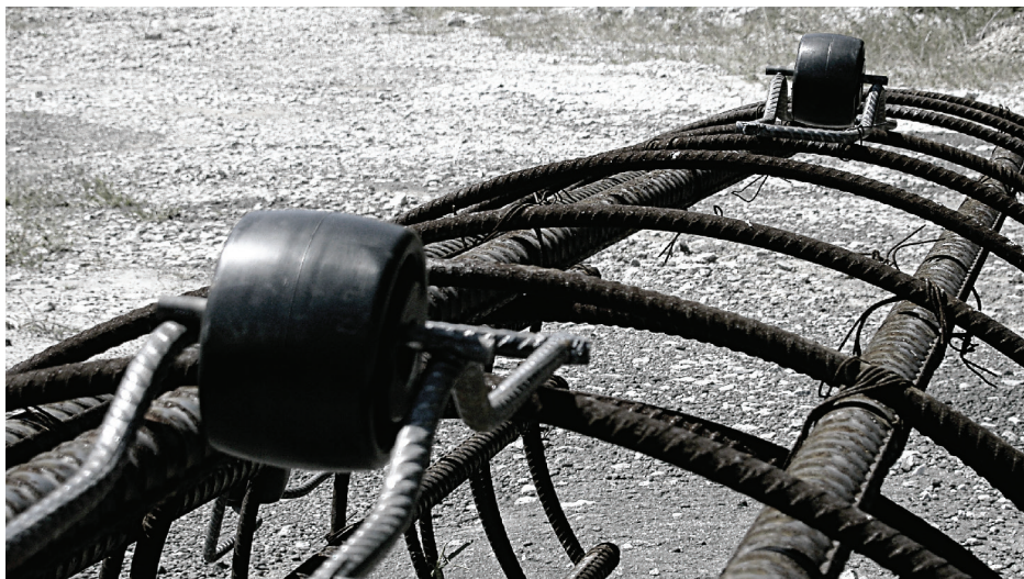
Reinforcement cage staged with Cagecasters attached for installation within battered shaft
