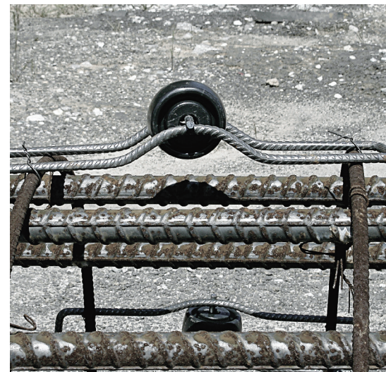
Cagecaster tied to horizontal reinforcement hoops
