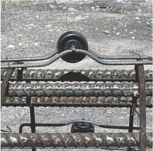
Cagecaster tied to horizontal reinforcement hoops
