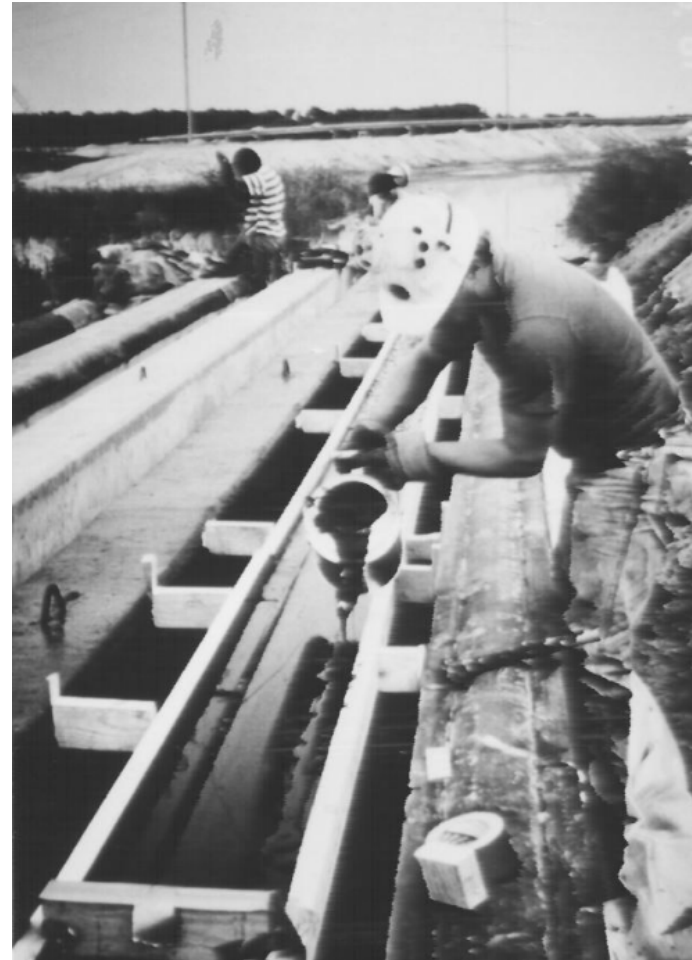
Applying the Bitumen:
