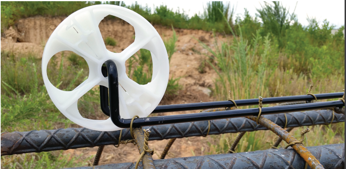
Attaching the Hairpin with tie-wire
