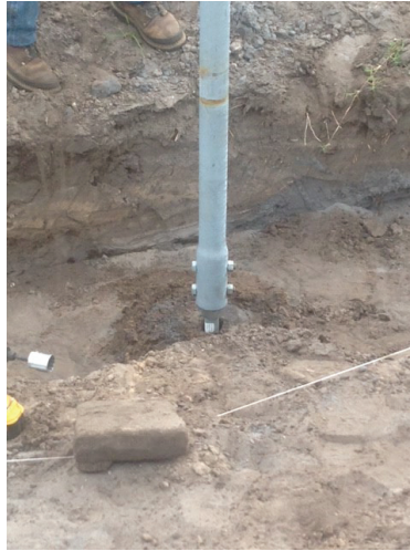
Square shaft to round connection
