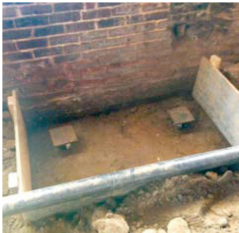
New construction caps set into new footing
