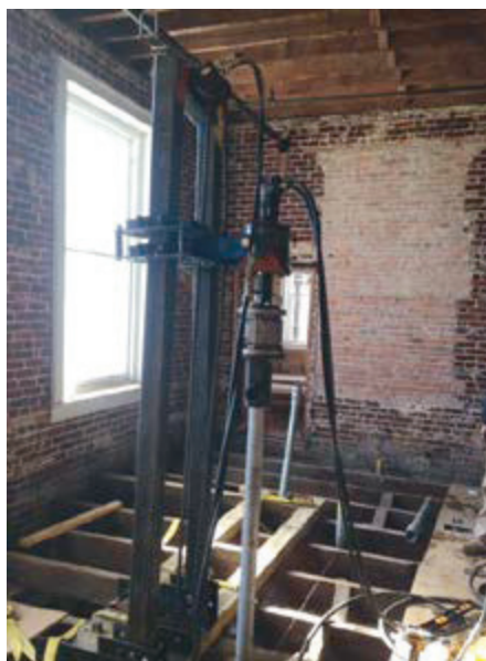
Custom mobile unit installing pile
