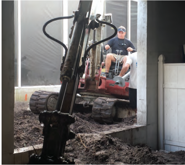
A HOLE WAS CUT THROUGH A GARAGE WALL TO PROVIDE ACCESS
