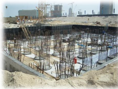
Pile trimming
