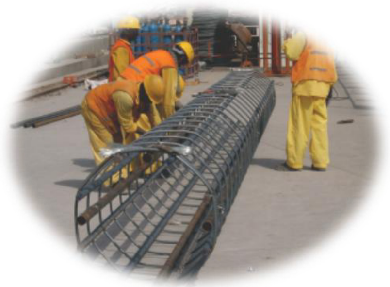
Sonitec tubes installation
